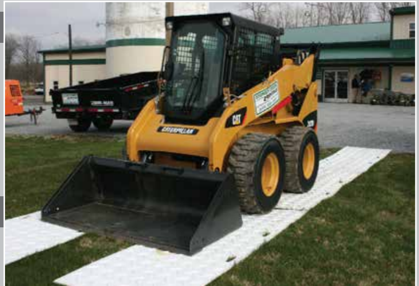
AM36 Mats locked together to form a continuous roadway
