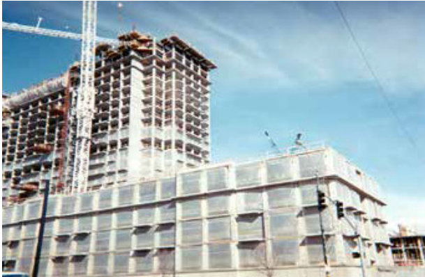
Building Abatement Enclosure
