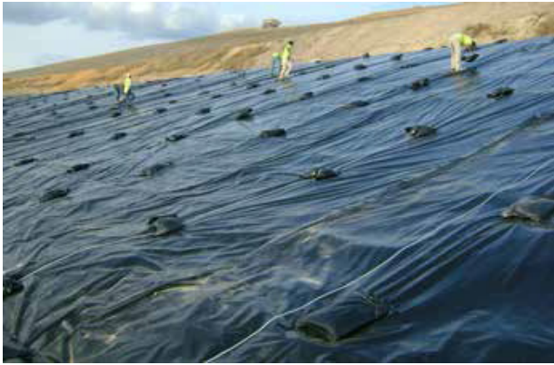
Temporary Rain Shed Cover
