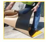
Easiest installation of any surface applied detectable warning. Just peel and stick, roll the mat to ensure a secure bond and install stainless steel anchors. Less than 10 minutes - start to finish.
